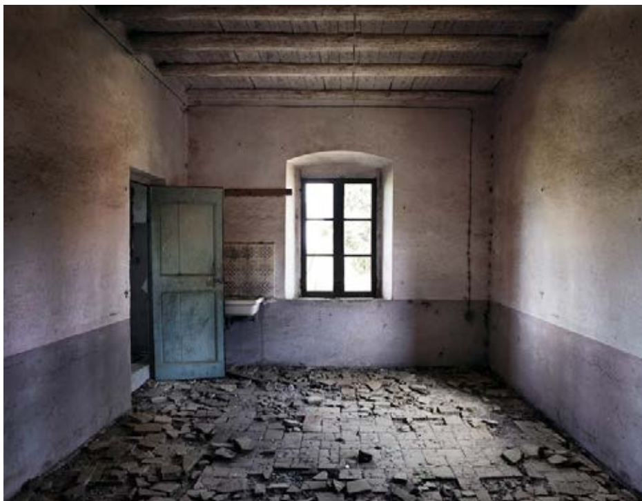
Marina Paris, Under construction
